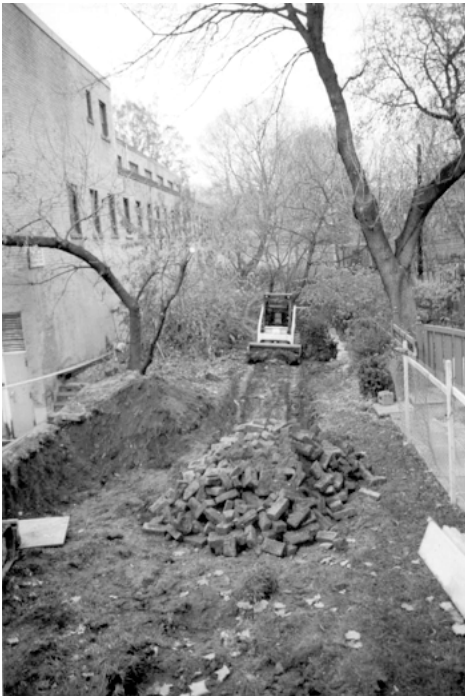
Site preparation revealing fill material.
