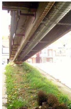
The umbilical cord bridge/walkway showing coupled sewage and water lines.
