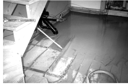
Radiant floor heating system under construction.
