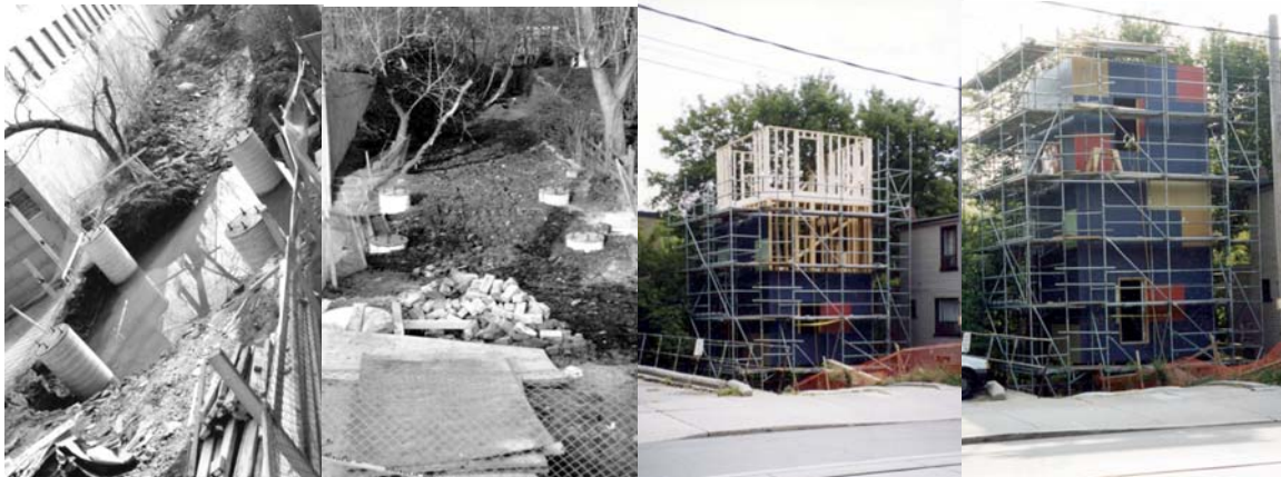
Left: Water emerges to the surface as the piles are being driven into the ground, showing the marshy nature of the natural soil condition. Filling the marshy soil. Right: Photos of the house at various stages during the six-months construction phase.
