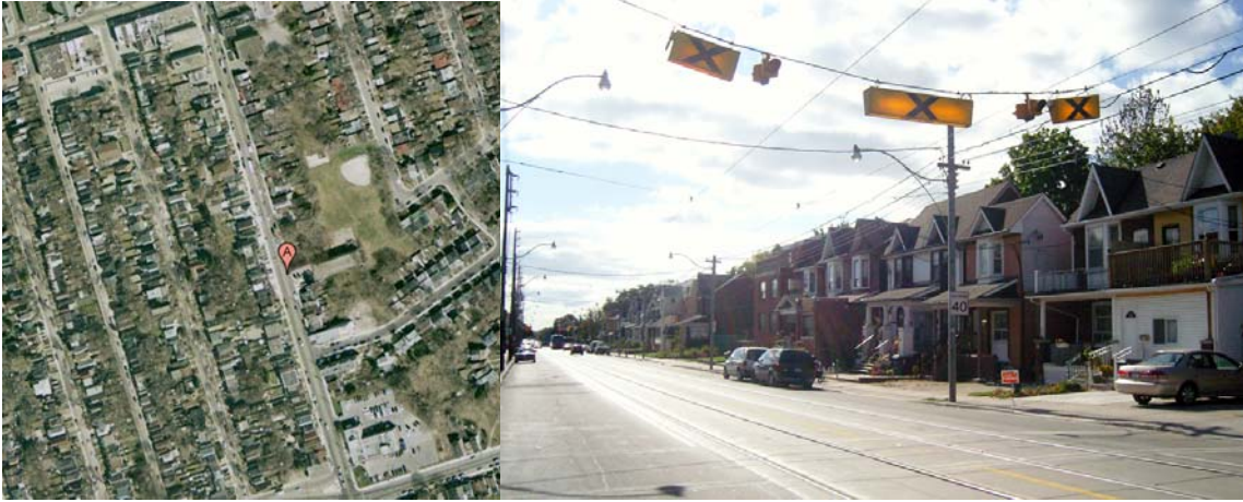
157 Coxwell House is located in Ward 32- Beaches-East York, Toronto. Looking South on Coxwell Street, showing homes on the West side, facing the Coxwell House.
