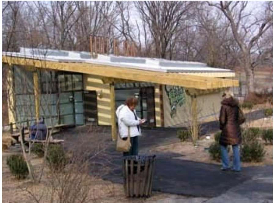
Bronx Zoo composting toilet installation / Image courtesy of www.treehugger.com
