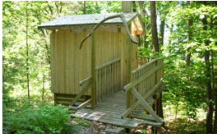
Photos left to right: The mixing tines in the interior of a Phoenix composting unit One of the composting toilet installations at St. Lawrence Islands National Park
